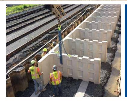
**T-WALL®** is a gravity retaining wall system, consisting of modular precast concrete units and select backfill. The system is a simple proven solution for grade separation on highway, bridge, railroad, water, commercial applications, and more.
