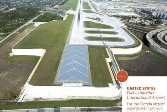
and more particularly for the extension of the south runway, Reinforced Earth designed and supplied 570,000 sq. feet of 62-foot high Reinforced Earth® walls.
