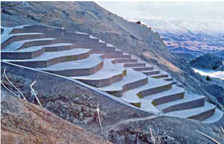
Stabilization of Landslide
