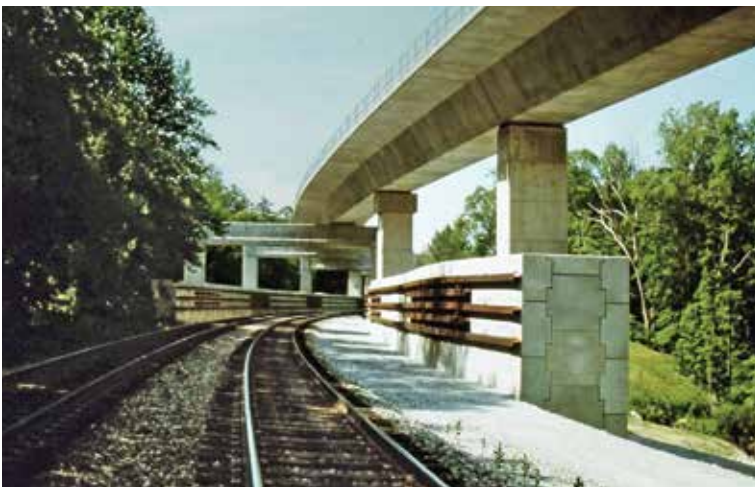
Deflection Walls, MARTA Bridge Piers
