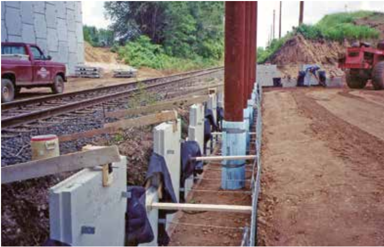
Concealed Crash Wall Construction
