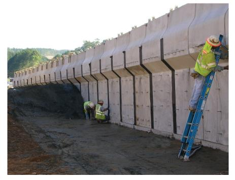
The primary components of a Piano Wall are full height precast composite MSE wall/traffic barrier units and alternating layers of granular backfill with high adherence, linear metallic soil reinforcing strips.
