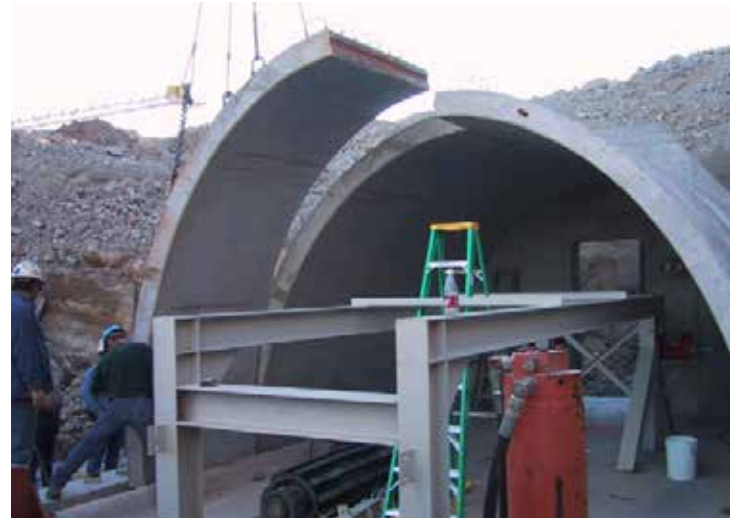
TechSpan Tunnel Construction
