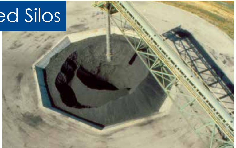
Reinforced Earth Inverted Silo
