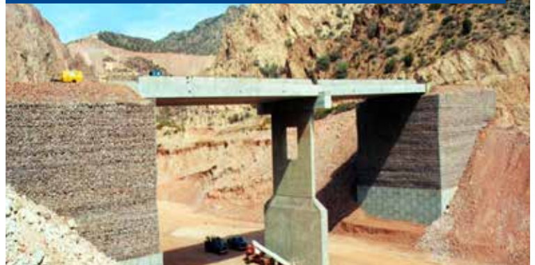
Haul Road Bridge Abutment
