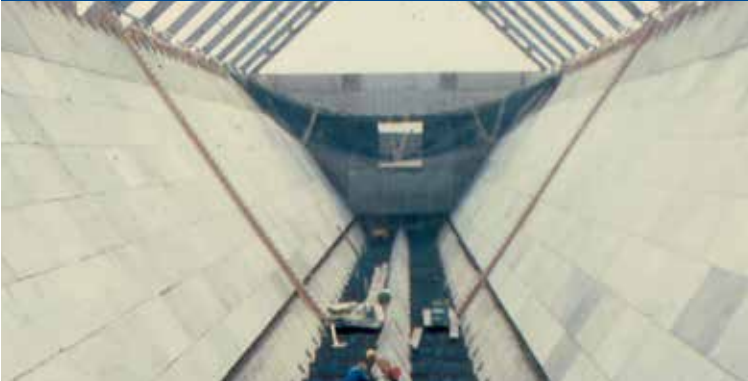
Reinforced Earth "V-Notch Slot"
