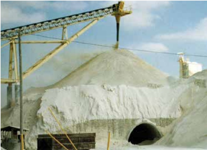
TechSpan Reclaim Tunnel with Reinforced Earth Headwall
