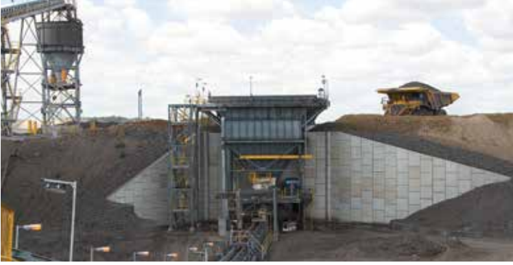
Reinforced Earth Crusher Pocket Walls
