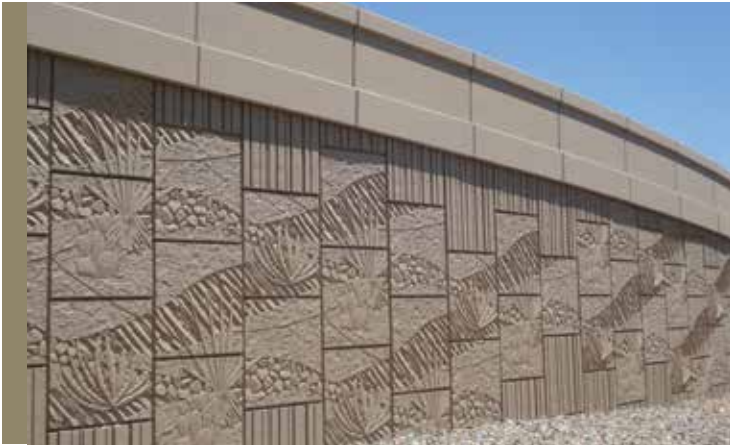
I-15 Design Build, Las Vegas, NV
