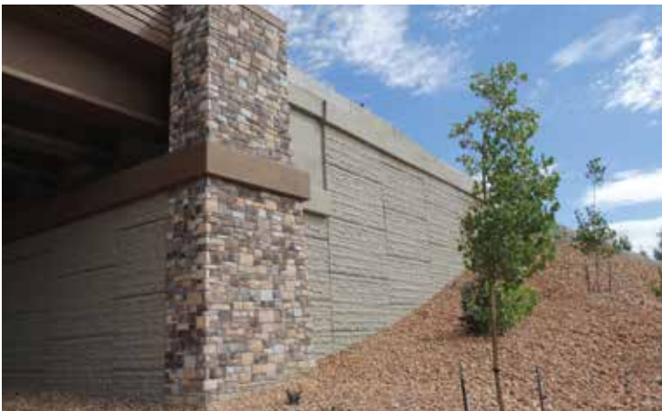
SR 92 Timpanogos Hwy, Lehi, UT
