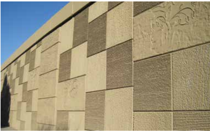
RTD West Corridor, Denver, CO
