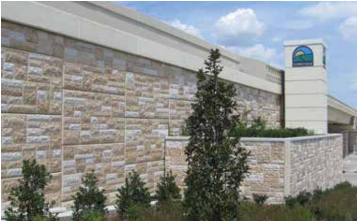
US 80 @ Collins Road, Sunnyvale, TX
