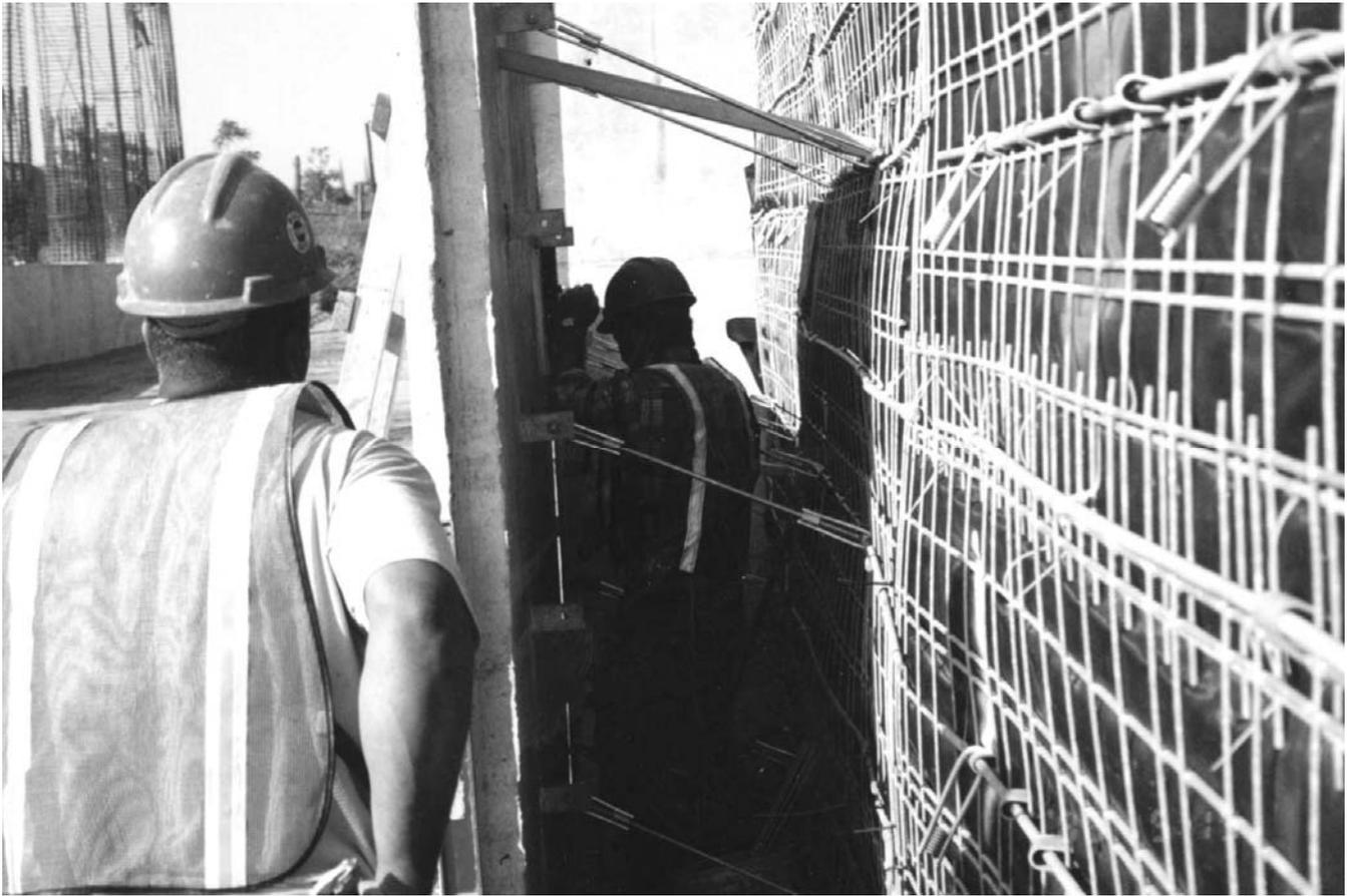
Figure 2. Connection of precast panels to wirewall.
