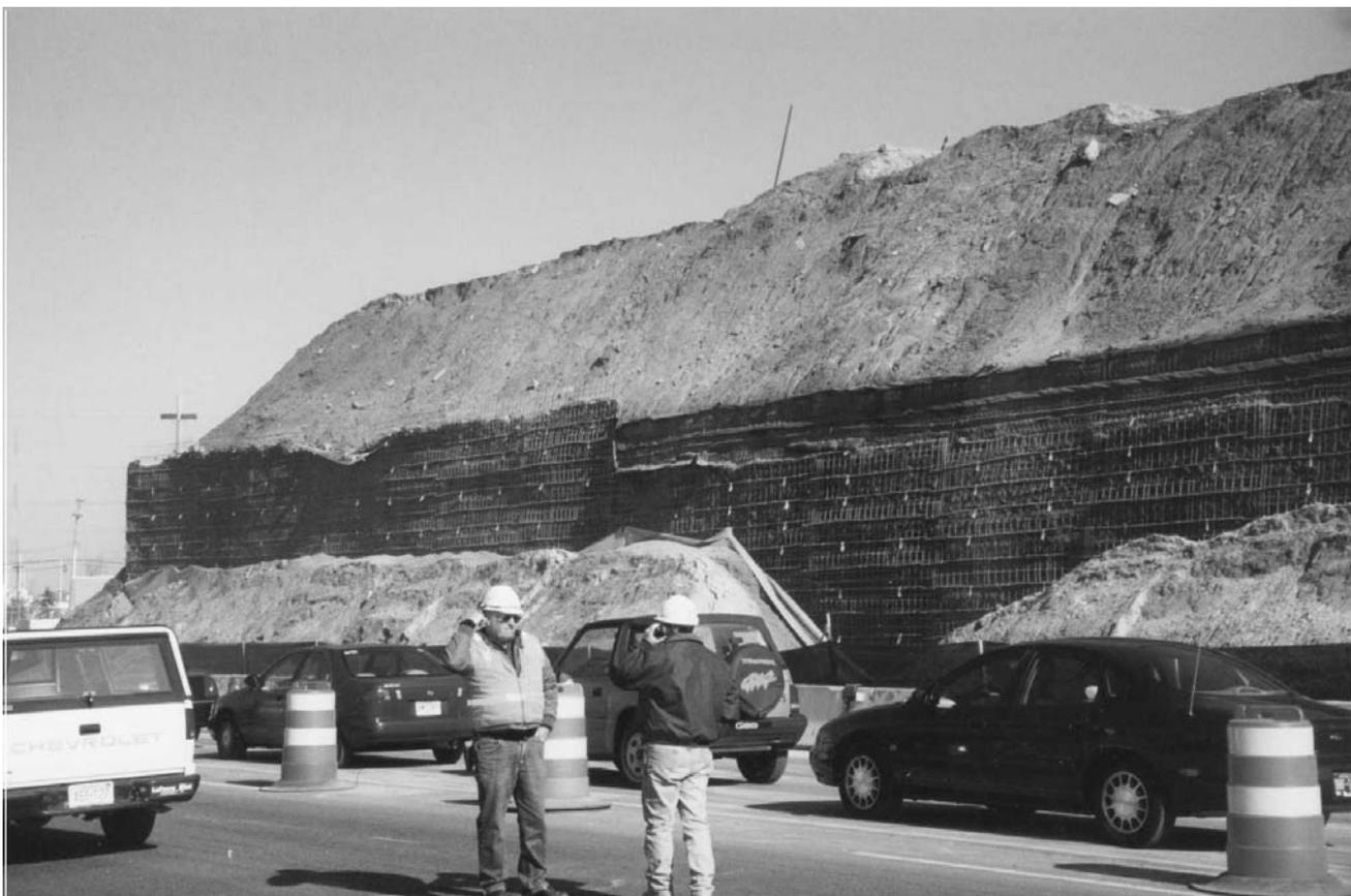
Figure 4. Temporary surcharge on wirewall, Atlantic City.
