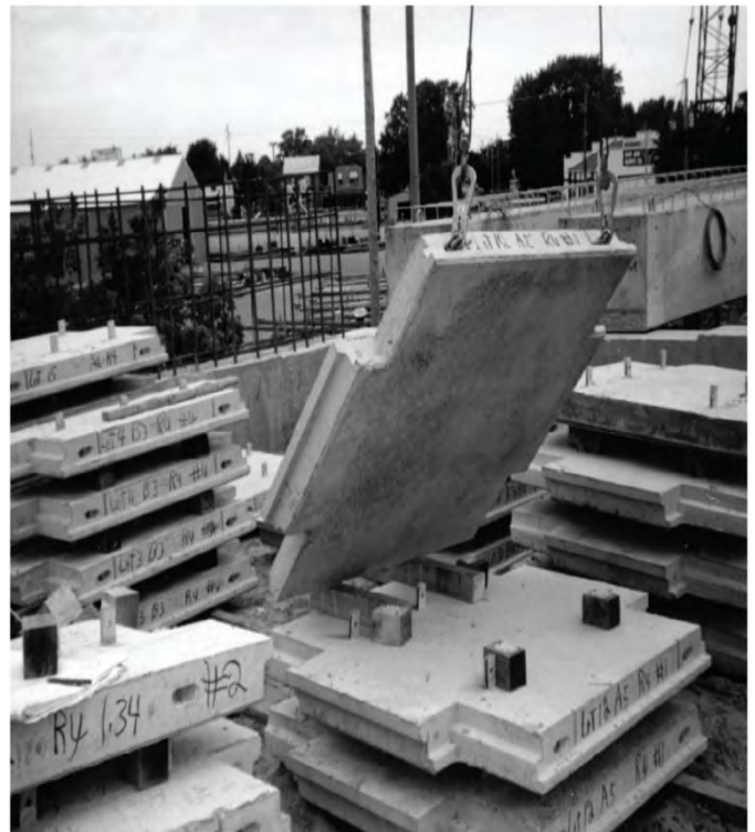
Figure 7: Lifting devices for handling individual panels.
