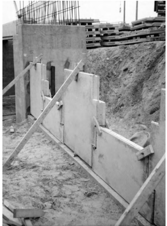
Figure 22: Braced initial course of panels.
