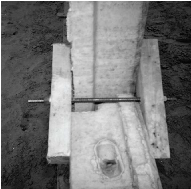
Figure 21: Panels secured with a clamp.
