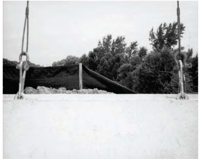
Figure 6: Lifting devices for handling individual panels.
